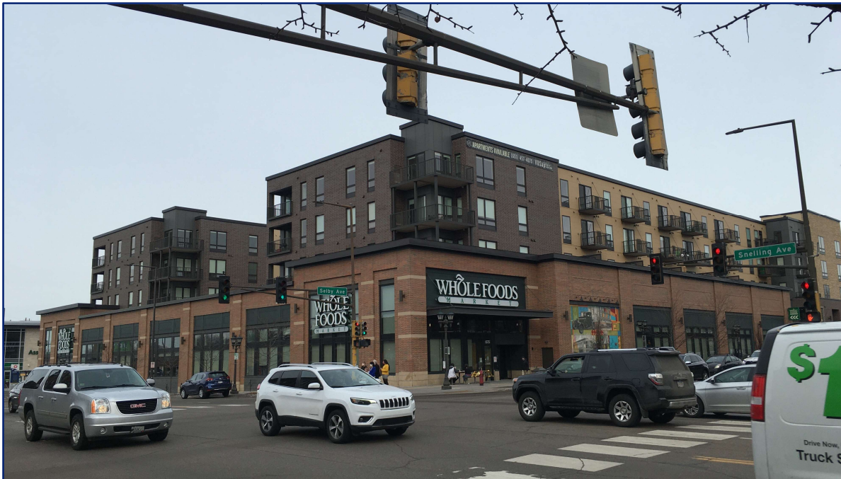
The Vintage on Selby, looking northeast
