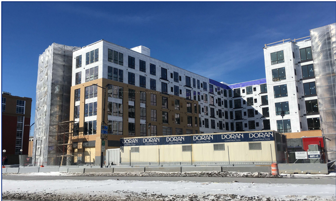
Mixed-use development under construction in downtown Saint Paul (not profiled)
